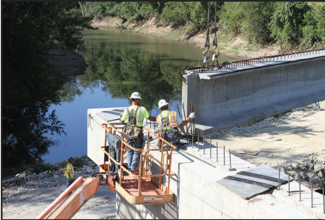
Figure 2. Bridge girder with instrumentation being set.
