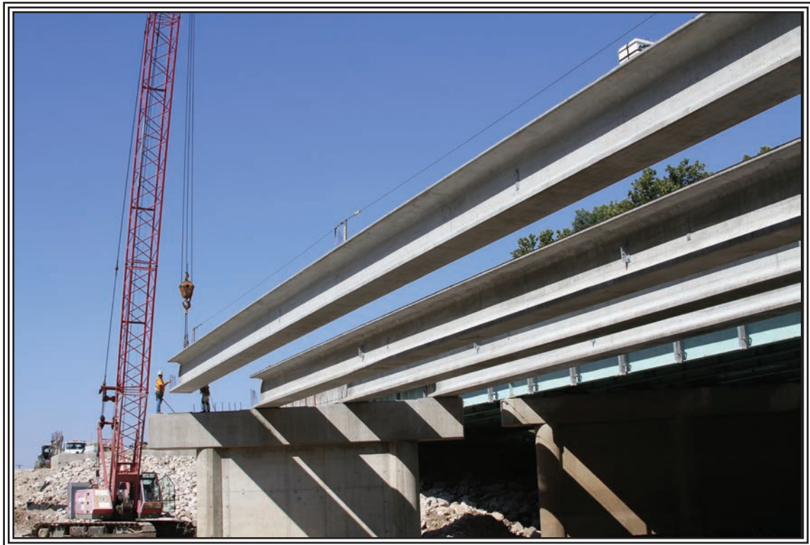
Figure 1. Final bridge girder for Span 2 with instrumentation being placed.
