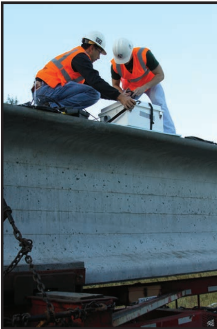
Figure 3. Missouri S&T graduate students Eli Hernandez and Alex Griffin attaching Data Acquisition System to bridge girder.
